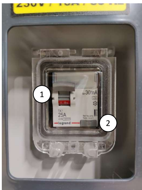
Figure 12. Residual current device
